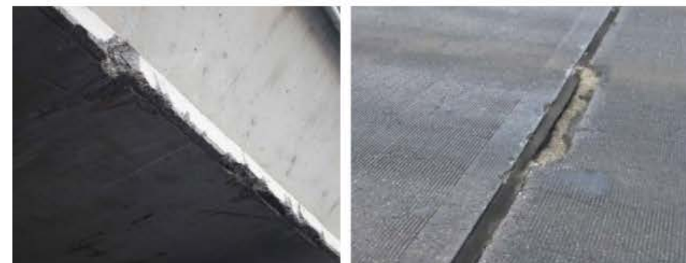
Signs of wear include spalling, cracking, and water intrusion.
